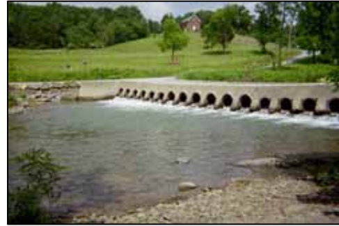
Fifteenmile Creek flows under this bridge built by WPA in the 1930s
