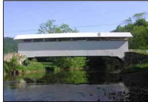
Hewitt Covered Bridge spans Town Creek
