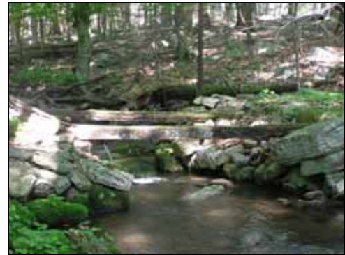
Old bridge abutment over Sweet Root Creek
